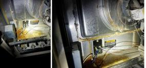
Manufacturer: Lennox Model Number: G40UH-48C-110-01 Serial Number: 5800K44851 Type: Forced air Capacity: 110,000 BTU Area Served: Whole building Approximate Age: 17 years Fuel Type: Natural gas Not Inspected Heat Exchanger: 5 Burner Marginal Blower Fan/Filter: Direct drive with disposable filter - Recommend changing furnace filter Acceptable Distribution: Metal duct Acceptable Flue Pipe:
